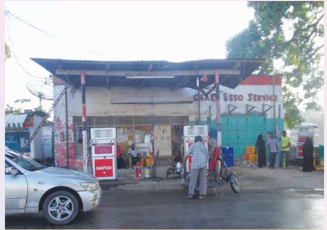
Kituo cha Chake Petrol Station kikionekana kabla ya marekebisho
